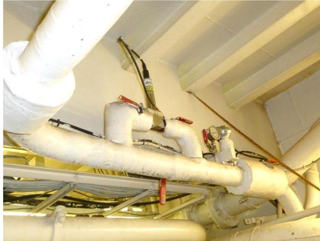
**Figure 24.** SBE38 temperature sensor in the engine room. This picture is from a previous year and during the winter refit 2016-2017 changes were made to the plumbing but essentially this is the same configuration.
