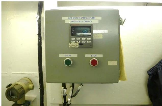
**Figure 23.** Honeywell controller for the pump, located in the TSG lab.
