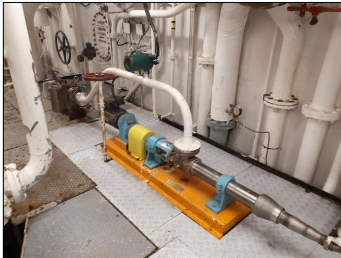
**Figure 21.** The Moyno pump installed in the engine room (2021).
