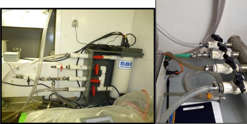
**Figure 20.** TSG manifold and water supply manifold ( 2019, similar for 2021).
