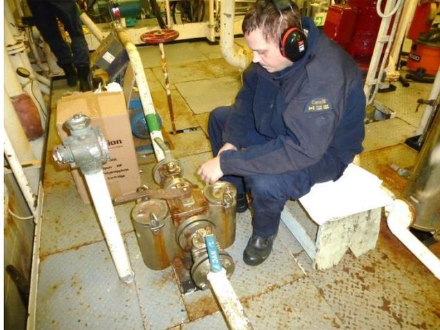
**Figure 22.** Seawater passes through a filter before going to the pump (in background). When the ship is in sea-ice the flow is switched from one filter to the other to allow the necessary frequent clearing out of slush from the filter. This picture is from a previous year but is the same strainer configuration for 2021.
