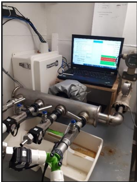
Figure A2. TSG manifold, flow meters, data logger and laptop (photo 2023).
