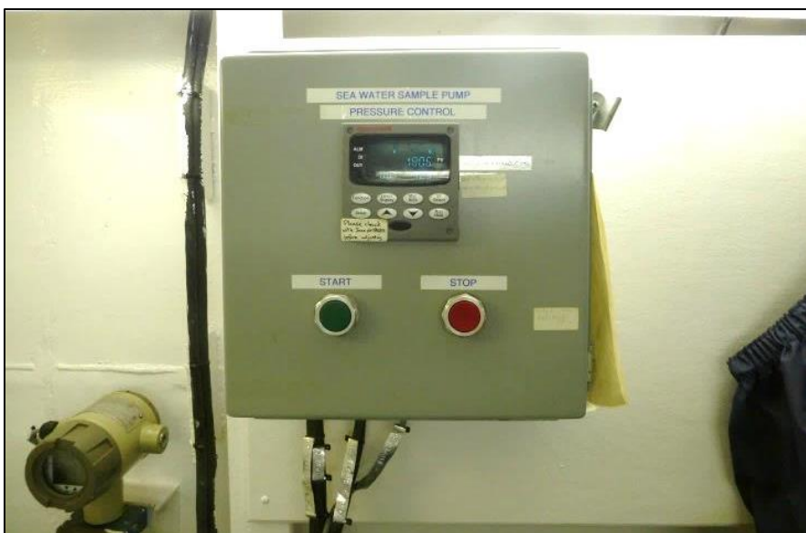
Figure A3. Honeywell controller for the pump, located in the TSG lab.
