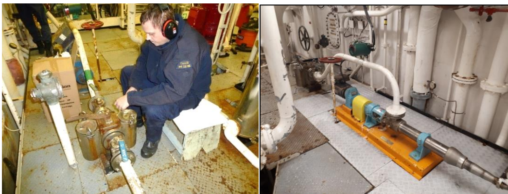
Figure A4. Seawater passes through a filter (in front of engineer) before going to the pump (on orange platform). When the ship is in sea-ice the flow is switched from one filter to the other to allow the necessary frequent clearing out of slush from the filter. Photos are from previous years, but is the same strainer configuration for 2024.
