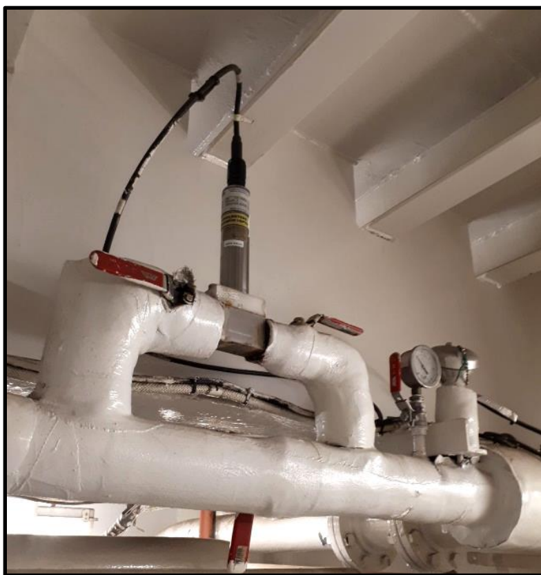
Figure A5. SBE38 temperature sensor in the engine room (2023). NOTE THE RED HANDLE AT BOTTOM OF PHOTO. THIS VALVE IS IN THE CLOSED POSITION DURING OPERATION. This handle is hidden from view when open, but needs to be closed to force flow past the temperature sensor to get accurate seawater measurements
