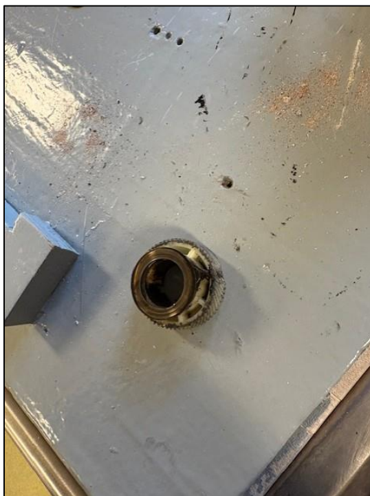
Figure 3.2.13-2: Image showing the stripped gear causing the issue with the pump.
