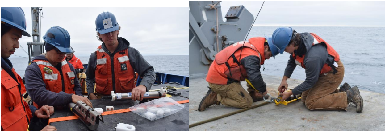
(left) Ray, Dan, and James replace microcat brackets on the fly. (right) Ray and Nico putting instruments inline on mooring deployment.
