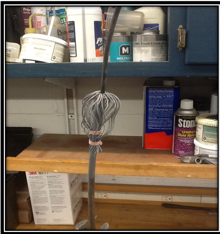
Cable ready to be pulled into termination
